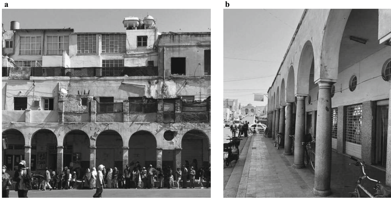
Fig. 6 a Asmara—Mixed-use building flanking the elongated marketplace (Author, 2022). b Asmara—The Colonnaded covered market along the North–South market axis (Author, 2022)
